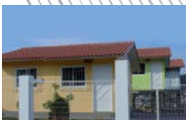
04 FRP panels Used the Construction of Brazilian Homes
