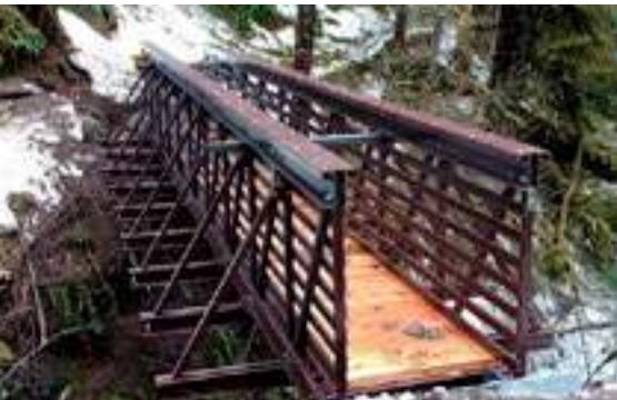
Cascade Locks, OR 40' span Shipped fully assembled
