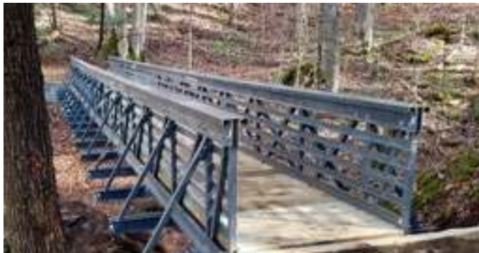
Banner Elks, NC 60' span Truss sections shipped assembled; other components field-assembled
