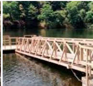
Cumberland Valley Township, PA 40' span Shipped fully assembled
