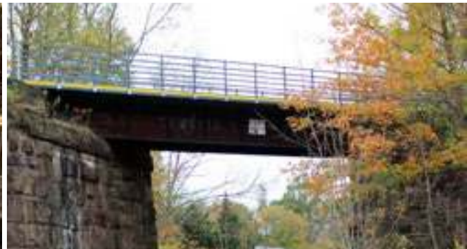
Johnstown, PA 190' span Shipped loose for field assembly
