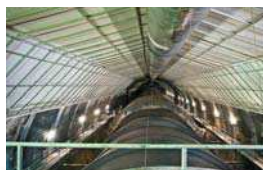
05 FRP Canopies Protect Steel Pipe in Hoover Dam's Penstock Tunnels
