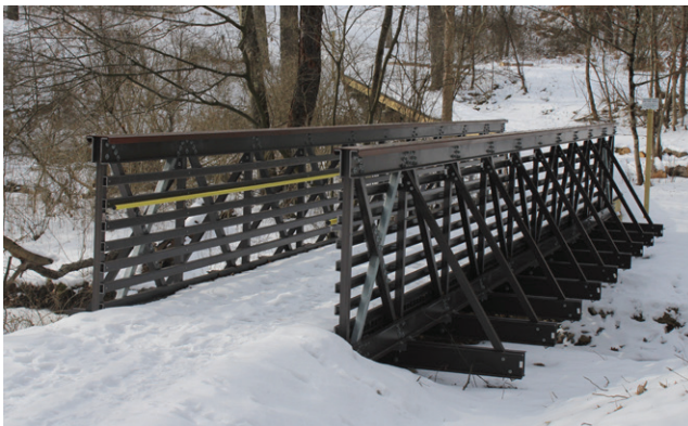
TRUSS BRIDGE WITH STRAIGHT END
