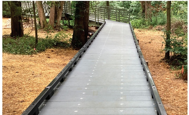
WIDE-FLANGE BEAM BRIDGE WITH CURBING
